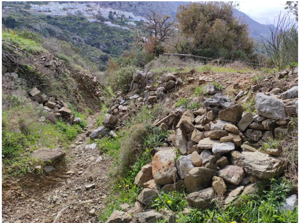
Picture 5: View towards the south before the works.
