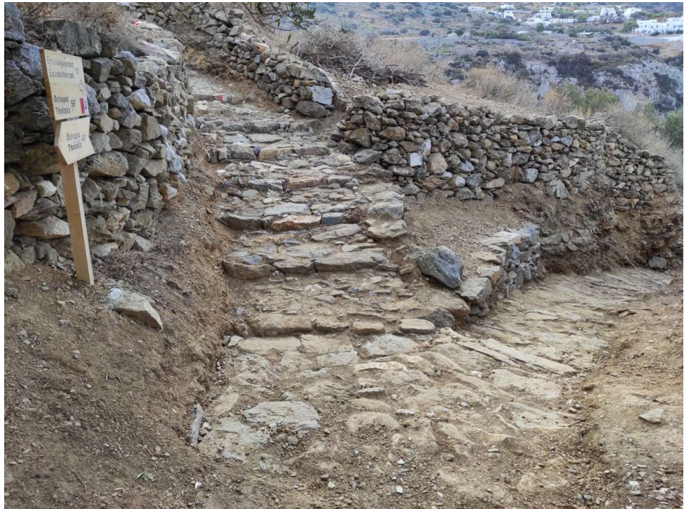
Picture 2: The intersection of path 4 after the works.
