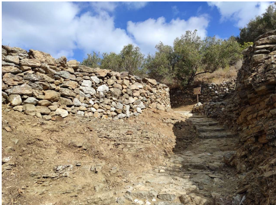
Picture 4: View towards the north after the works.
