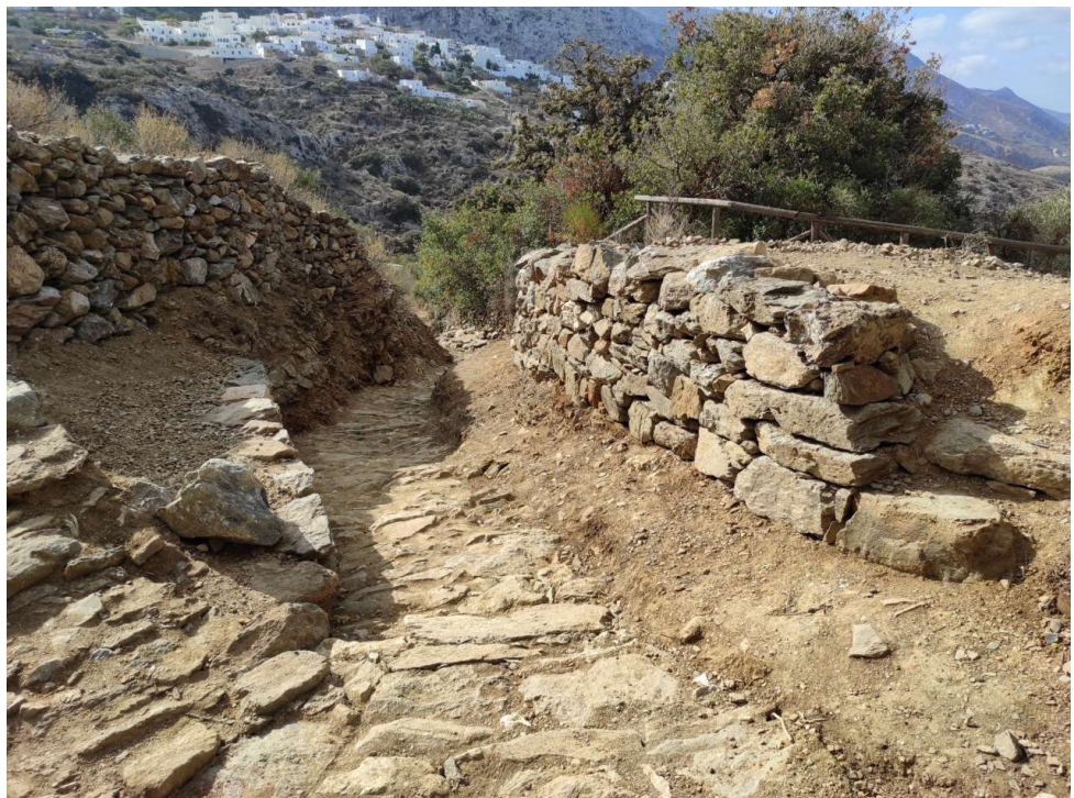
Picture 6: View towards the south after the works.
