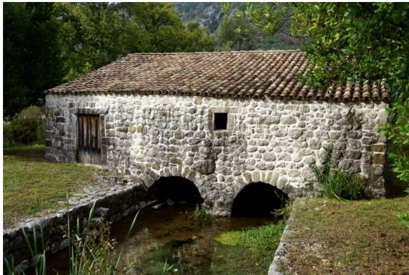
p 4.18: The chutes over the mills are very narrow, but the water released after the millwheels flows in a wide riverbed. The millwheels can be seen in the corridorspace deep under the mill building (Ljuta river 2021).
