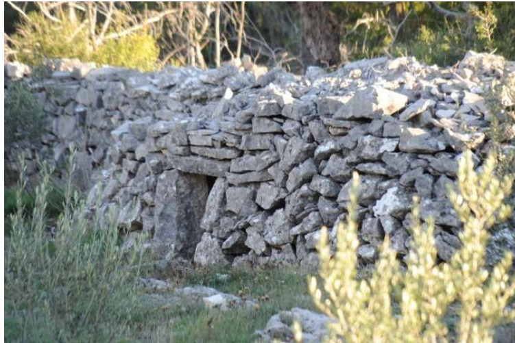
p 4.15: Only a few objects in stone can be found in Herzegovina today. This poljarica is incorporated into a wall, but it is large enough to protect stool as well as some people in the case of sudden rain.
