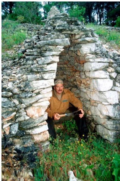
p 2.1: Corbelling in principle appears as cross section: it can compose a room as longitudinal construction, in space it is false dome, with circular ground plan. This simple shelter has a seat for one man only, trim on island of Hvar, Croatia.
