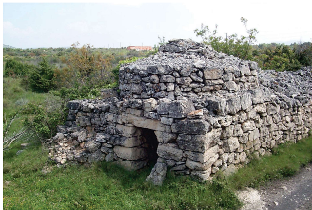
p 4.6: An interesting combination of a square ground plan and circular rings over it confirms its construction.
