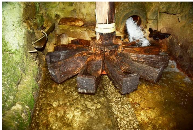
p 4.19: The waterwheel is made of very hard wood. Constant moisture is needed for a long lifespan. The paddles are designed for the best effect, but are simplified because of the simple carpenter's tool. This wheel can be seen in the cold stream under the last watermill (Ljuta 2021).
