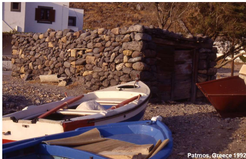
Fig.4: The stones found in each area and dry stone technique were used to build a variety of constructions, and even huts sheltering small fishing boats on the coasts of numerous islands.
