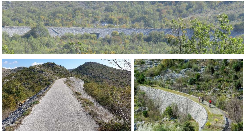
Figures 14.-16. Monumental dry-stone embankments of the Gabela-Zelenika railway on the Zaplanik-Uskoplje section, Ravno Municipality, with culvert and cantilever steps (above) and in locality Bijela (bottom, left); Bicycle path along the old railway route (bottom, right) 20
