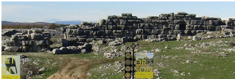
Figure 3. Daorson walls whose construction is based on the weight of carved bunny blocks and precise processing of adjacent surfaces, which allows better bonding and earthquake resistance
