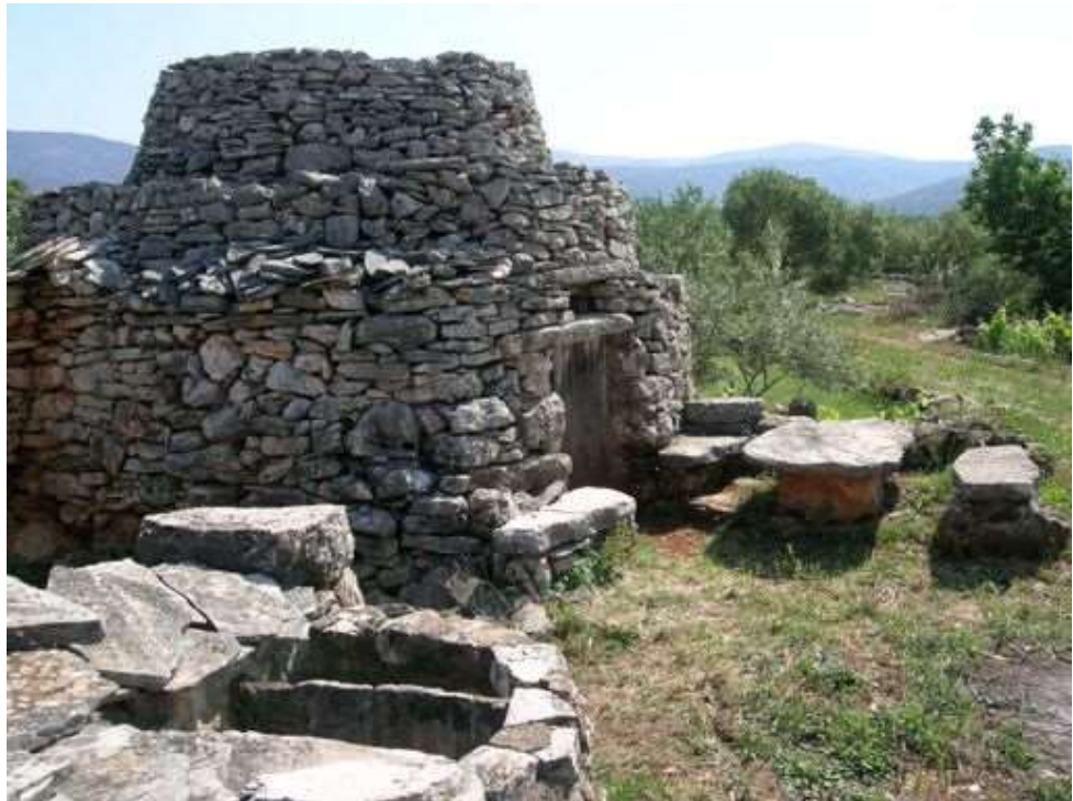
Picture 16: Distinctly elegant example of corbelled dry-stone shelter, trim, Stari Grad Plain. © Berislav Horvatić
