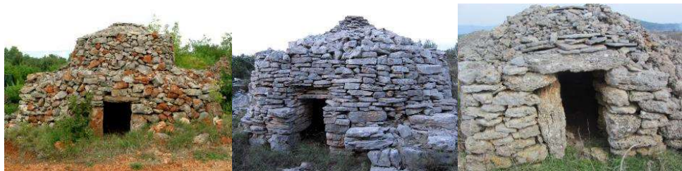
Picture 17: Examples of various rock types used for constructing trimi on Stari Grad Plain, ~1960. © DGU
