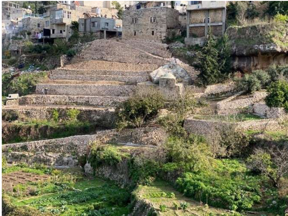
foto 2 =newly constructed drystone walls in Palestine
