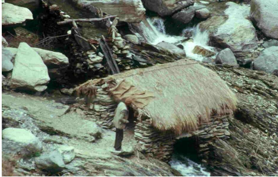
Figure1 water mill fed by dry stone lined water channels alone. (no backing)
