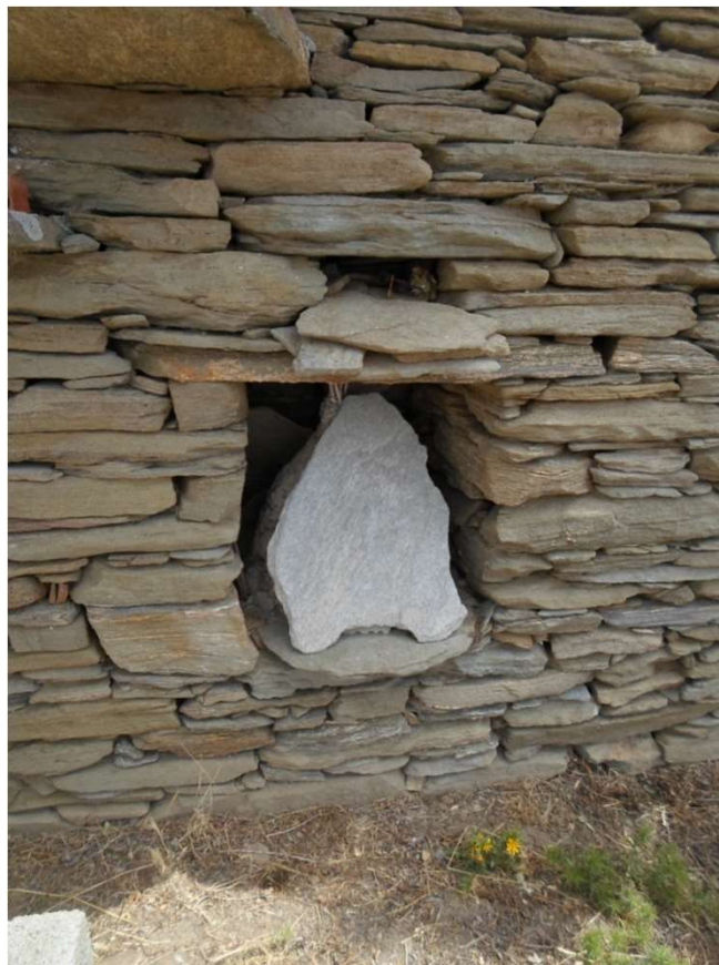
Fig. 2 Bee hole with upright wicker skep, protection stone slab, and “polemistra” at the bee entrance.
