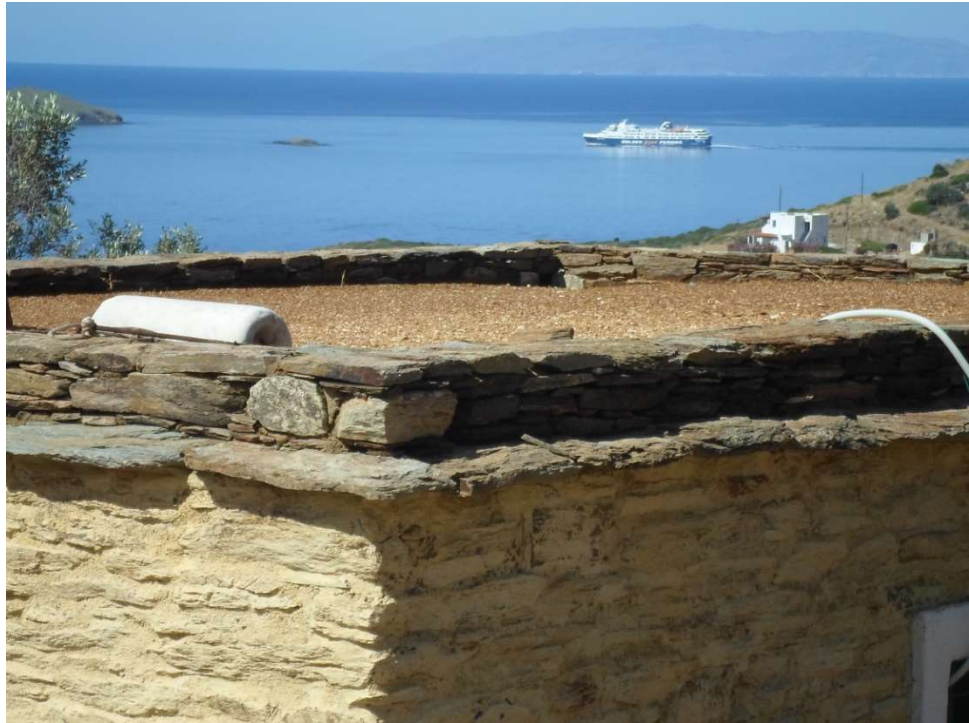
Fig. 10 Rehabilitated bee house at Kipri, which is now used as office. On the roof a cylindrical marble block that is used for the maintenance of the roof.
